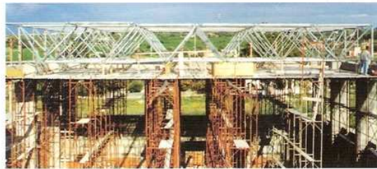
Erection on scaffolding, Catania Sports Hall / Italy
