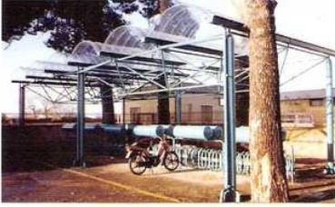
Rome Railway Canopies / Italy
