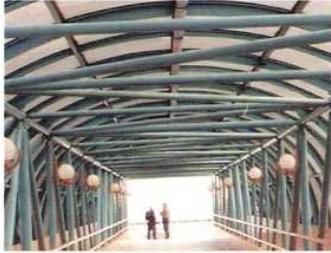
Samatya Pedestrian Overpass-Istanbul / Turkey Curved arch purlins system
