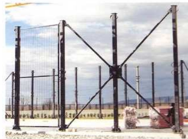
Otokar - Land Rover Plant Structural Steel Framing / Turkey
