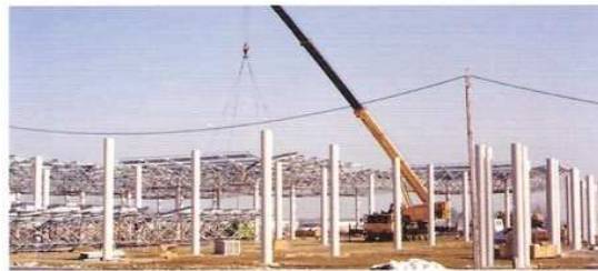
Erection by crane, Cuneo Market Hall / Italy
