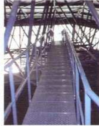
Kazan Universal Sports Hall Catwalk system / Russia
